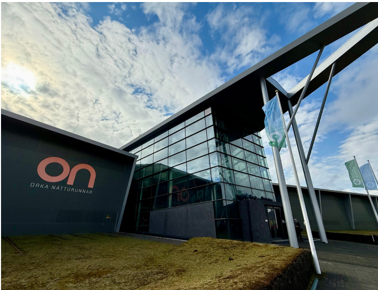
Hellisheiði Power Station
